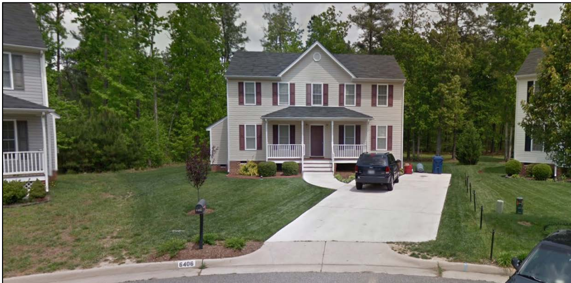
Figure 3: Street view of 6406 Bareback Terrace
