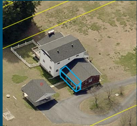
Existing Covered Walkway
