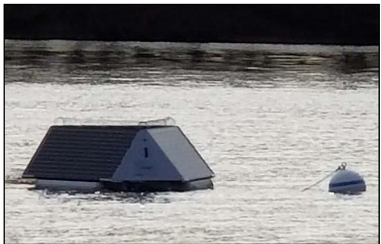
*One of two buoys located in the water treatment plant intake bay. Approximate dimensions are seven feet by eight feet wide and three feet high.*
